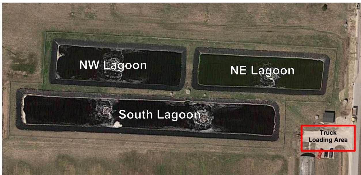
Figure 2-2: Essex-Windsor Solid Waste Authority RLF Site - Lagoons
