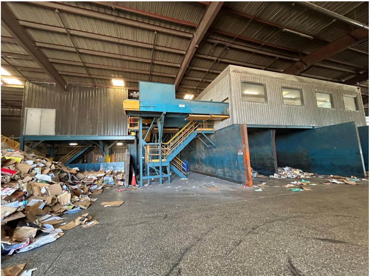
Fig 2.3- Left to right: fibre optic compressor room, pedestrian stairs, and second floor sort room
