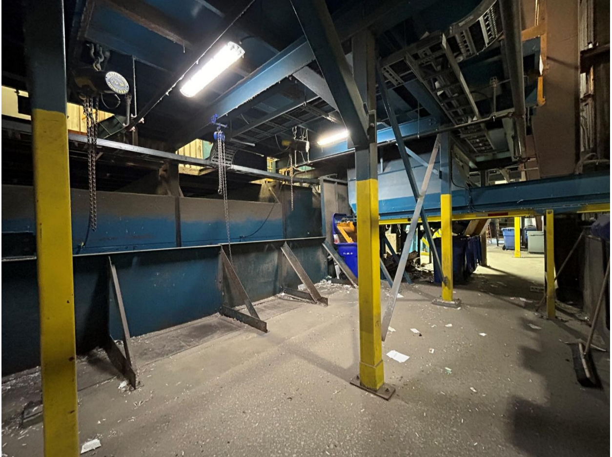
Fig 2.11- North bracing under Optic Sorter and mezzanine
