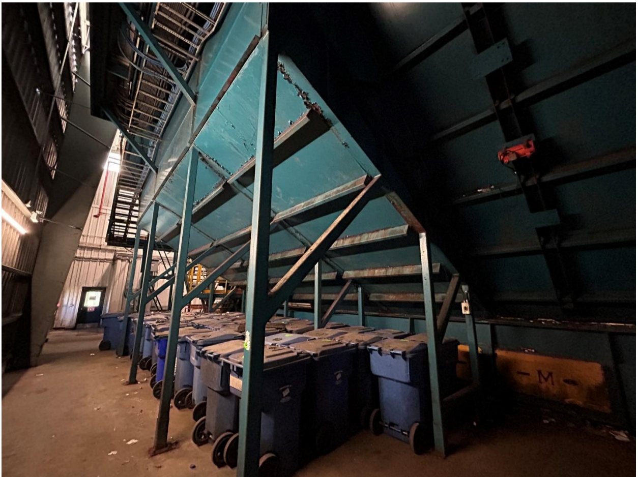
Fig 1.15 – Bracing under north portion of sort room and processing equipment
