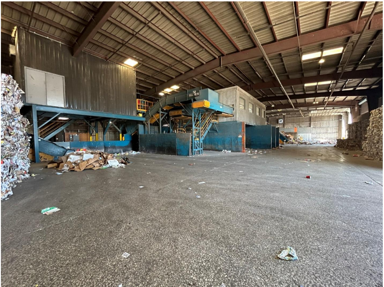
Fig 2.5 – Southeast overview of compressor room, stairs, sort room
