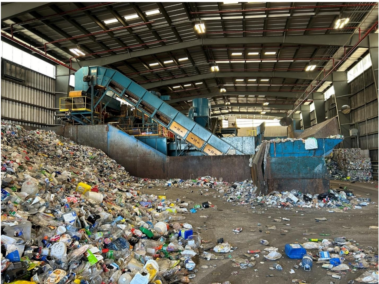
Fig 1.1 – MRF tip floor and west portion of hopper and sorting equipment
